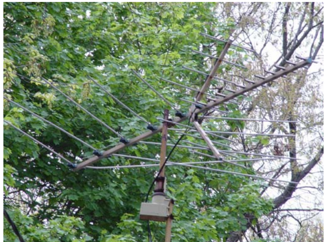
TYPICAL ROOFTOP ANTENNA
